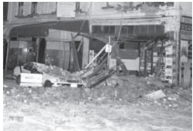
Some effects of the Christchurch earthquake
